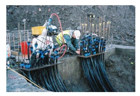
Figure 4 Flushing and pressure testing individual heat exchangers, National Assembly for Wales (Cardiff, Wales).
