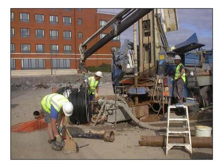
Figure 3 Drilling and installation of a vertical borehole heat exchanger, National Assembly for Wales (Cardiff, Wales)
